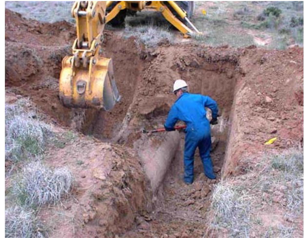
Excavating the 30 in diameter pipeline
